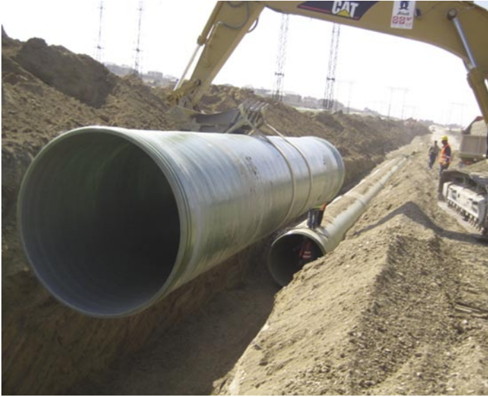
The low weight of the GRP pipe reduces the size of the lifting equipment required, lowering installation costs.
