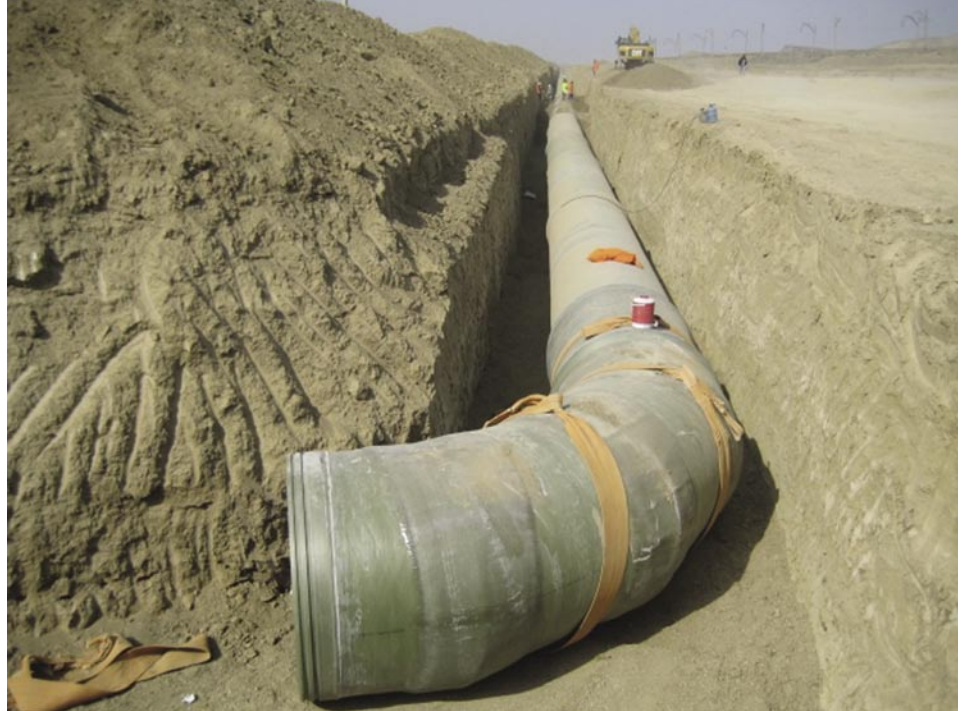
Each section of pipe is 12 m long and the pipeline will require 25 000 joints.
